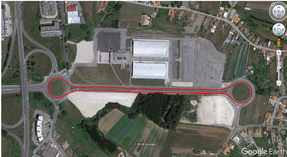
Fig. 6.38: Section of the road that was the subject of the study done for the case of the application of deep learning methodologies (marked in red in the image). This section generated 1070 frames processed by these two methodologies.
